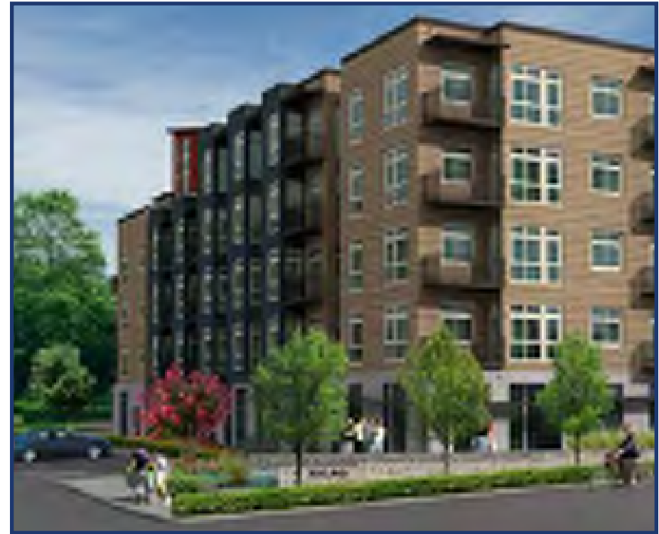
FIGURE 4-14: Malmo Apartments, Shoreline
