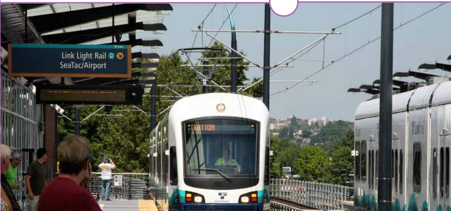
Link Light Rail Station
