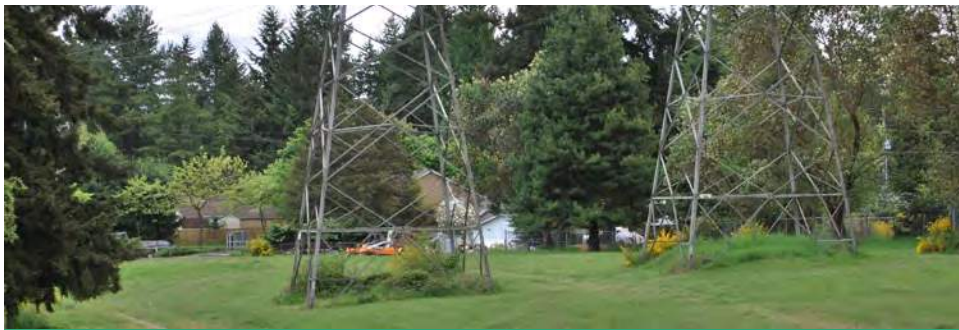
Seattle City Light Corridor
