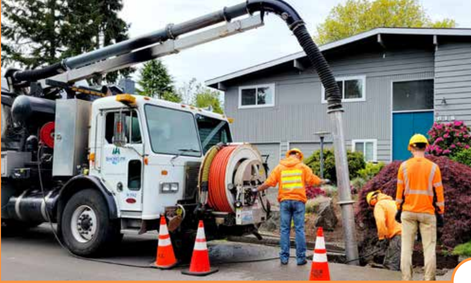
Maintenance workers replacing city facilities
